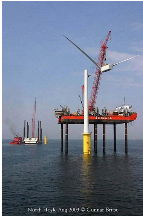
Figure 2.11: Installation using Jack-up vessel
