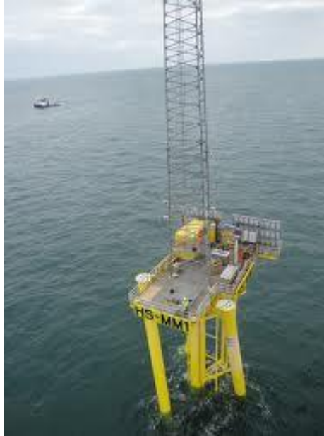
Figure 2.9: Hornsea Met Mast supported on Keystone “twisted jacket” structure ( www.smartwind.co.uk )
