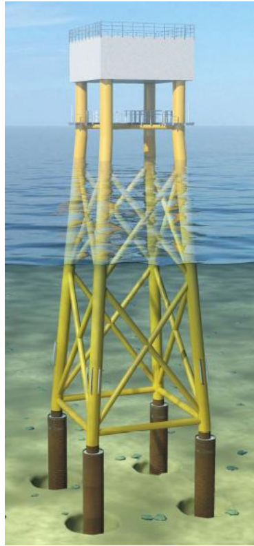
Figure 2.10: Jacket Structure (source Jensen 2010)
